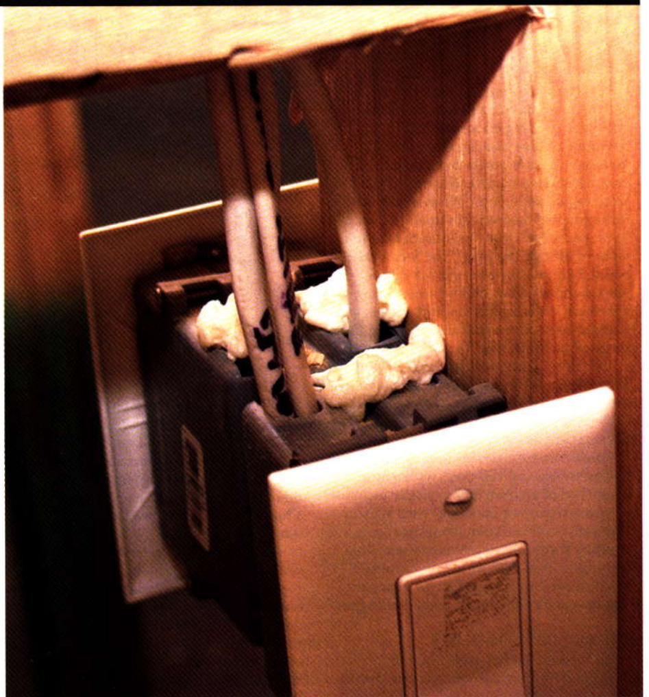
Proper sealing and insulation play an important part in engineering an airtight building envelope. These practices reduce heat flow and ensure a home will receive maximum benefits from energy-efficient features.
